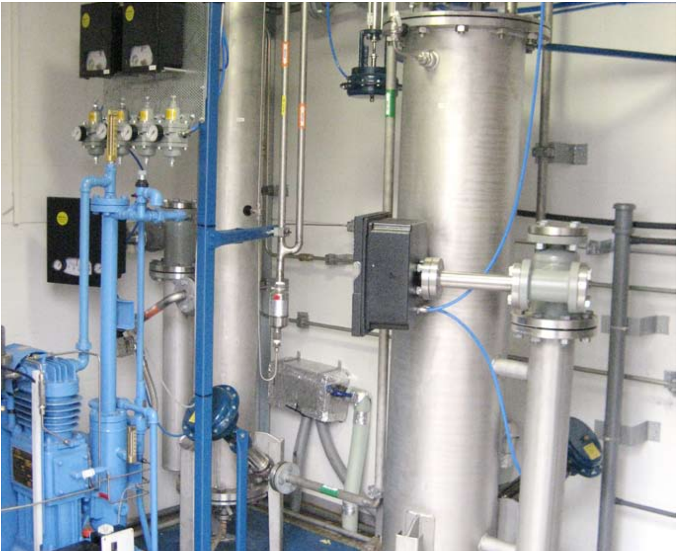
Upgrading biogas facility at biogas plant
