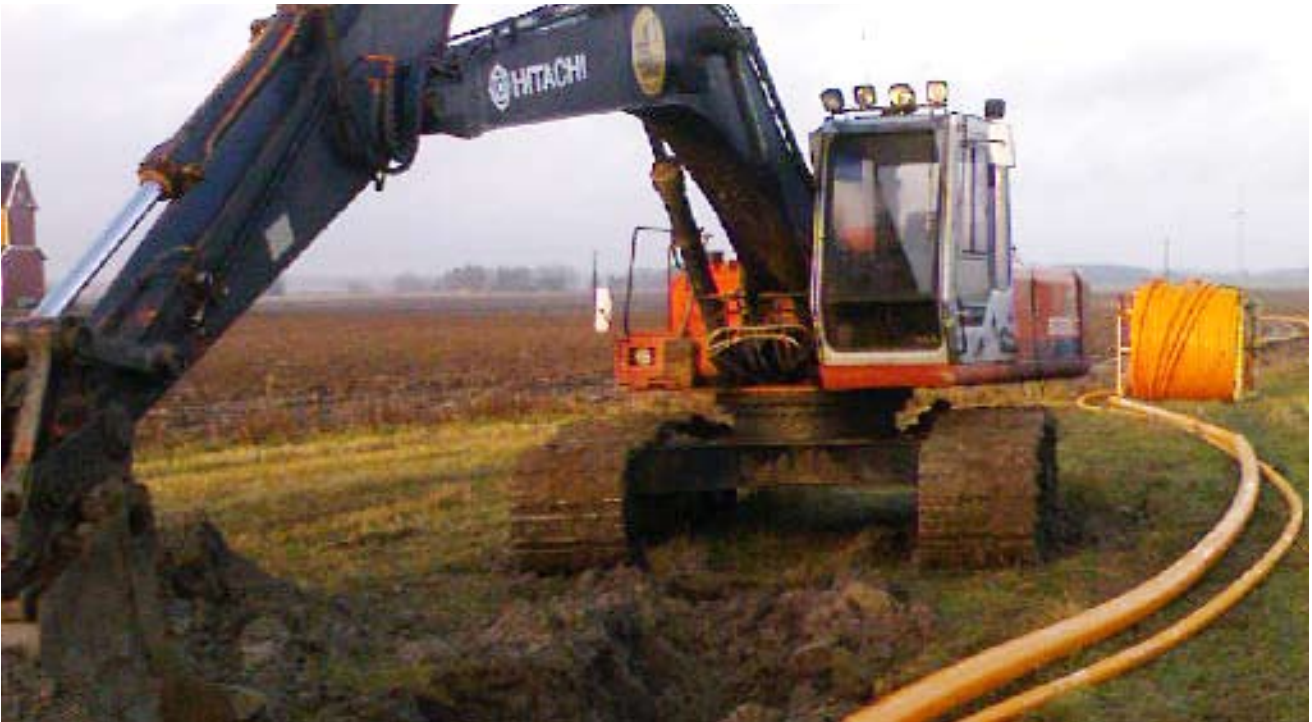
Laying down biogas pipeline in Fyrbodal
